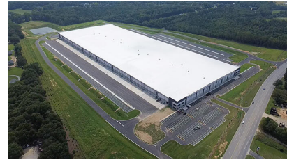
Exterior of new production facility (image courtesy of Colliers International)
